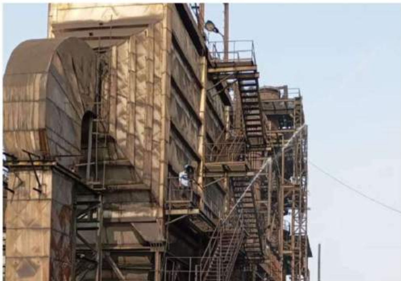
WATER SPRINKLER INSTALLED FOR FUGITIVE DUST CONTROL
